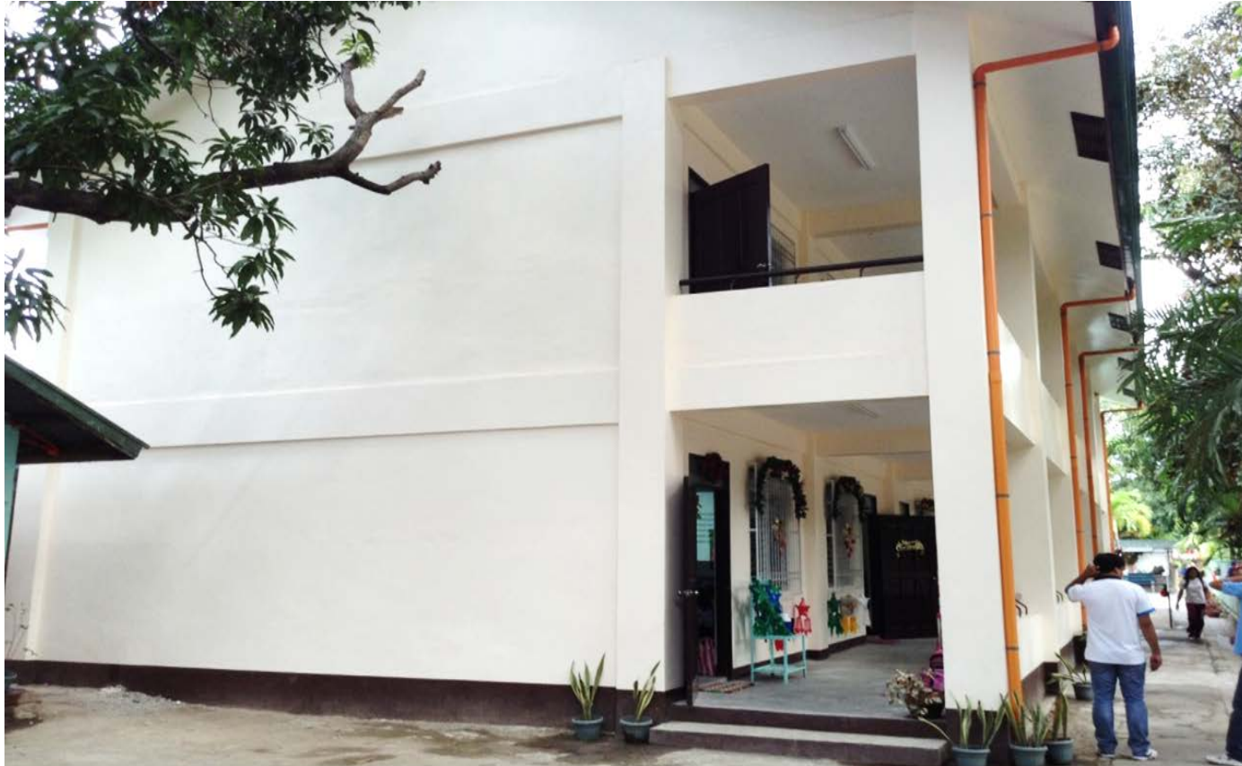
Two-Storey 4-Classroom School Building
